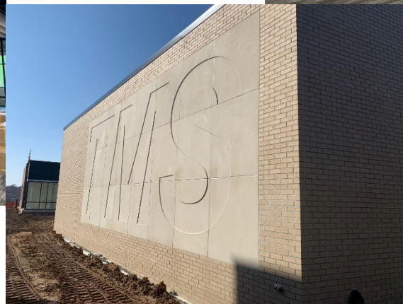
(left) Site work has started around the cast stone mural.
