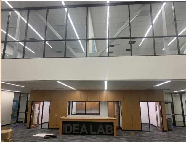
(below right) Idea lab casework and wood paneling is installed.
